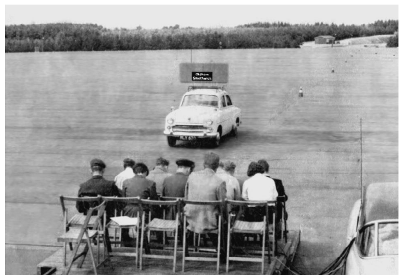
Figure 6. 'The experiment was greatly speeded up by mounting the signs on a vehicle and driving them towards a group of 10–15 stationary observers seated on a tiered platform.' Note the 'margins' of the board on which the signs are mounted. The subjects in the experiments were Royal Air Force volunteers, at Benson airfield, Oxfordshire. (Christie and Rutley 1961a, figure 4. The photograph was published in Christie and Rutley 1961b, p. 242, as figure 4; and later published in Mijksenaar 1971, p. 30.).
